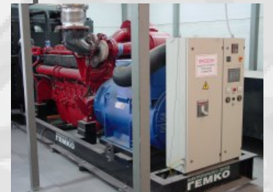
Emergency Stand by Generators 1500 KVA
